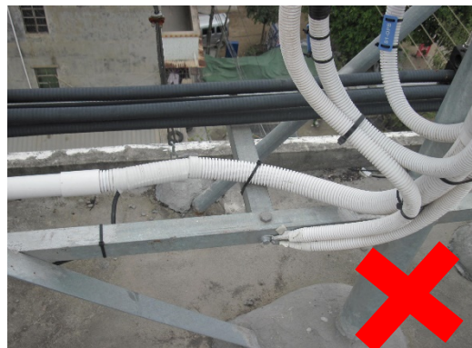
Disordered wiring of distribution box
