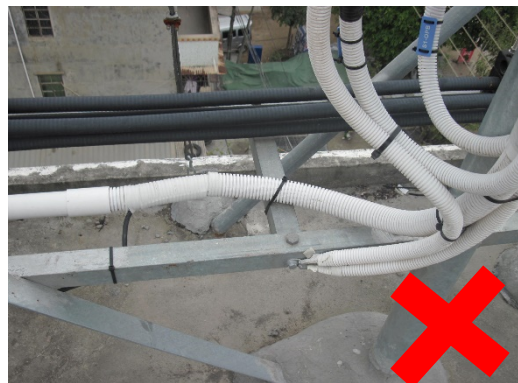
Disordered wiring of distribution box
