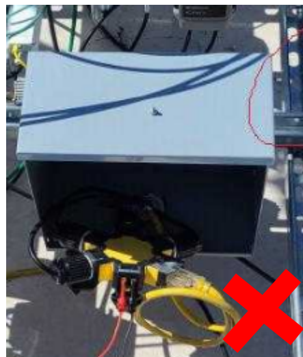
Disordered wiring of distribution box
